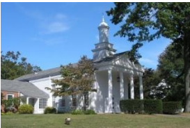
First United Church of Christ (Plymouth Building), 18 West Main Street
